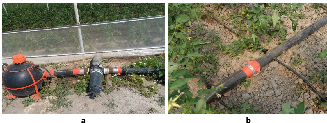
Figure 6. a Drip irrigation system. b Main and lateral pipes
